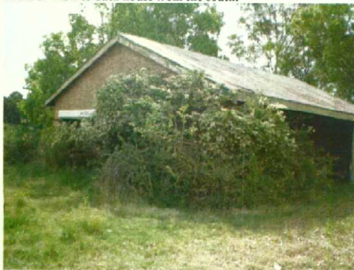
Photo 4 The bicycle shed at the rear of the bath house.
