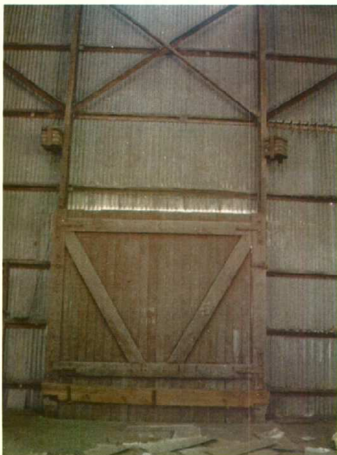
Photo 6 The original doors on the north wall of the store
