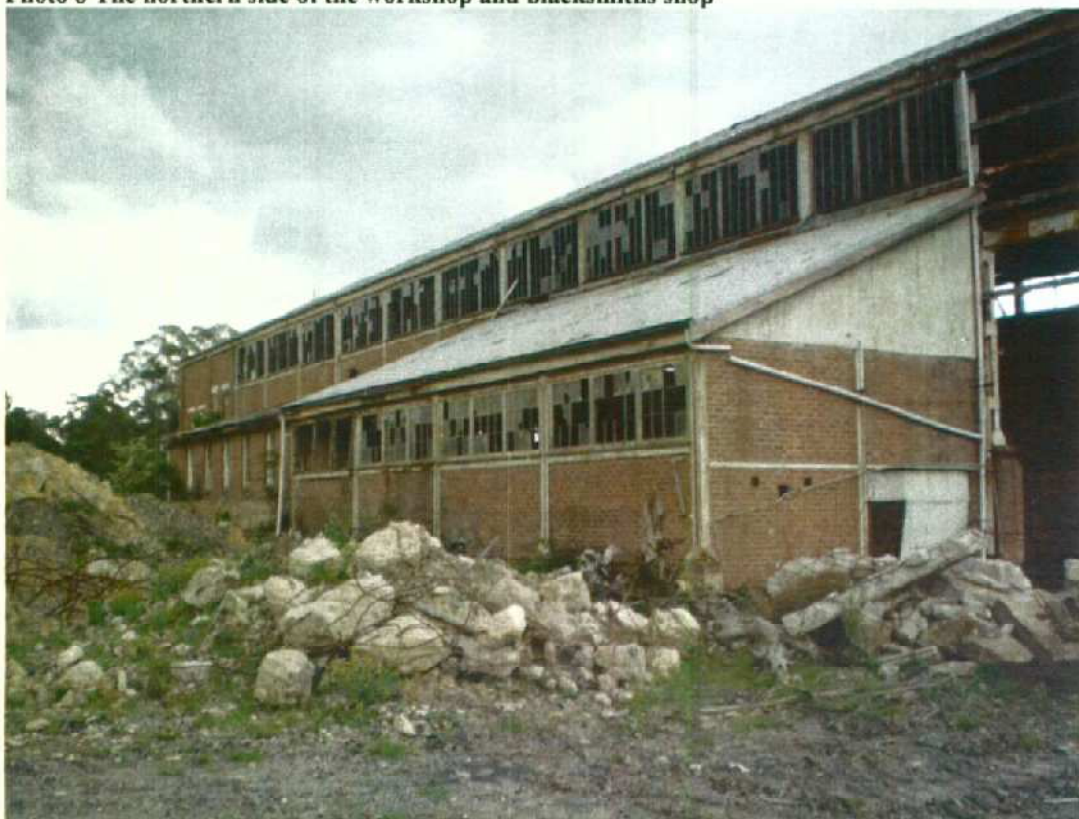
Photo 9 The southern side of the workshop and carpenters shop. Note open eastern end of building
