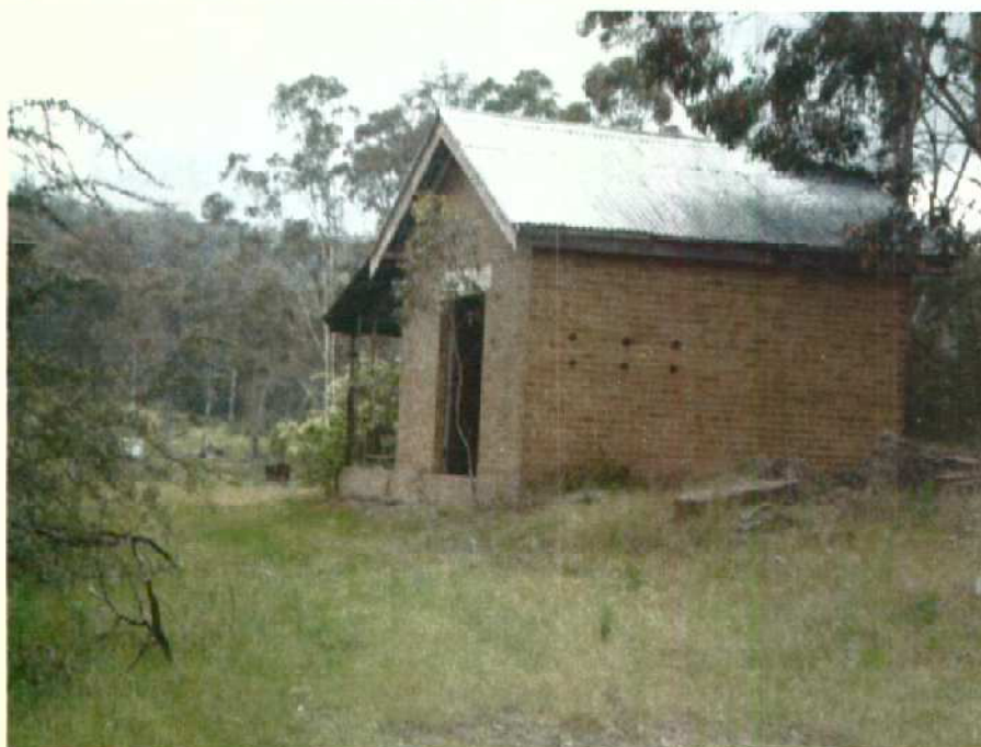
Photo 14 The fuel store at the rear of the engine house
