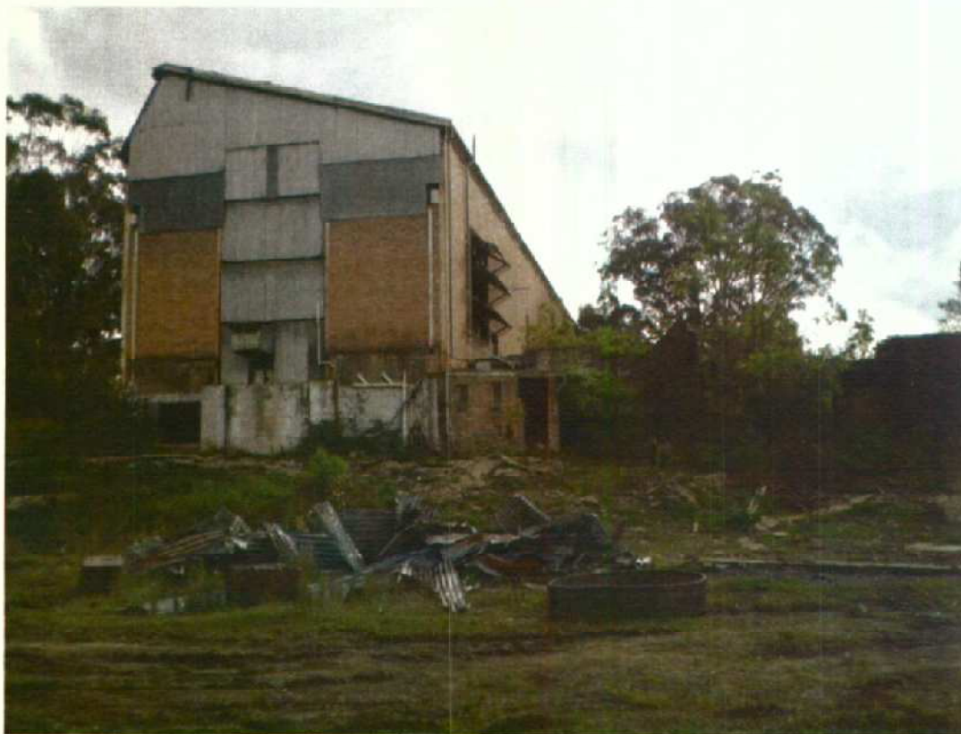
Photo 13 View of engine house from the east.
