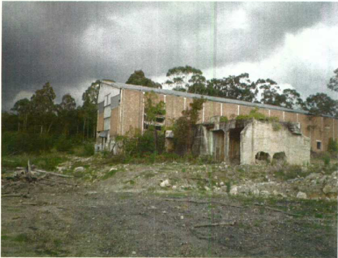
Photo 15 View of the engine house from north east.
