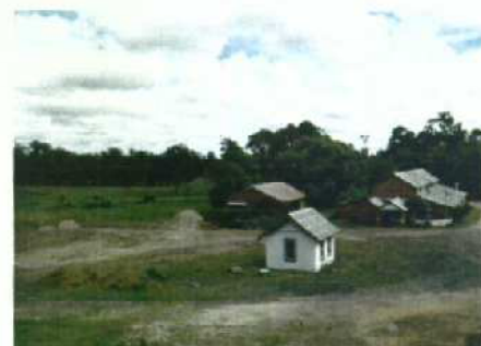
Photo of Subject Site
