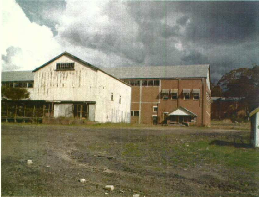
Photo 5 The Workshops with store at front, offices on the right rear, workshop left rear.
