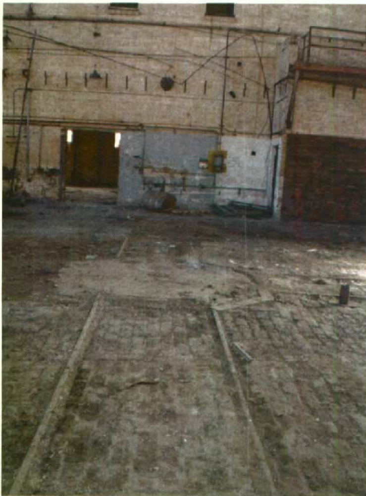
Photo 11 The light rail and turntable inside the workshop connecting to the store on the right. This feature can be conserved in an outdoor area attached to the office.
