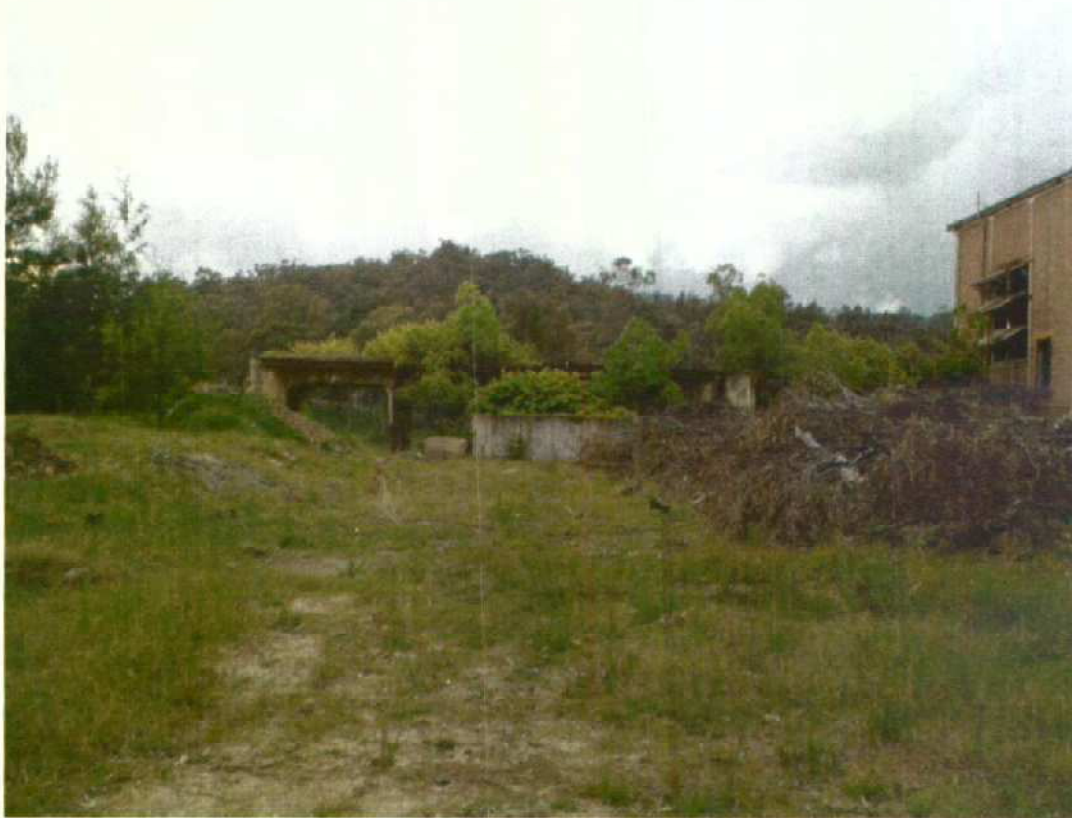
Photo 12 Remains of the overhead light rail structures and No. 2 shaft
