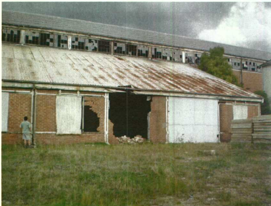
Photo 8 The northern side of the workshop and blacksmiths shop
